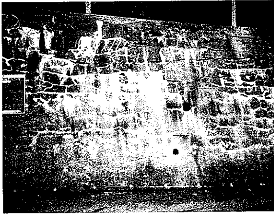
Photo 1 Damage due to alkali-aggregate
