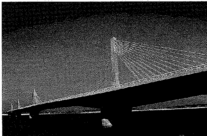
Photo 1-1 Completed KISO River Bridge
