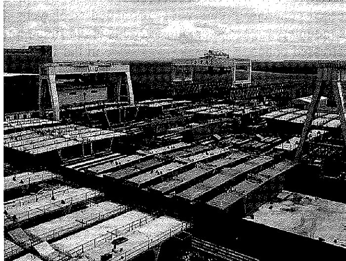
Photo 1-5 Prefabrication casting yard
