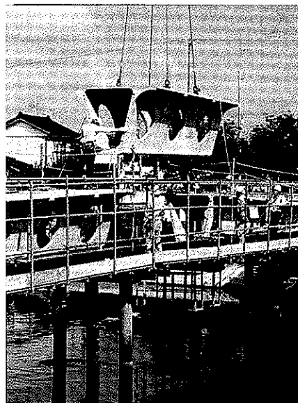
Fig. 41 Installation of block
