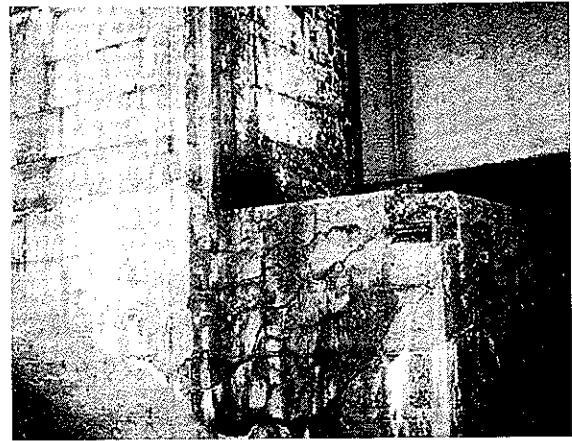
Photo 1 Damage due to alkali-aggregate
