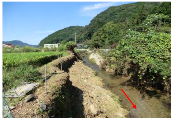
(c) 地点②での護岸の破壊
