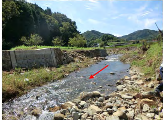
(c) 地点⑥での護岸の破壊
