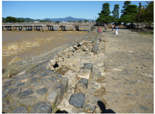
(b) 渡月橋右岸上流域の護岸の破壊
