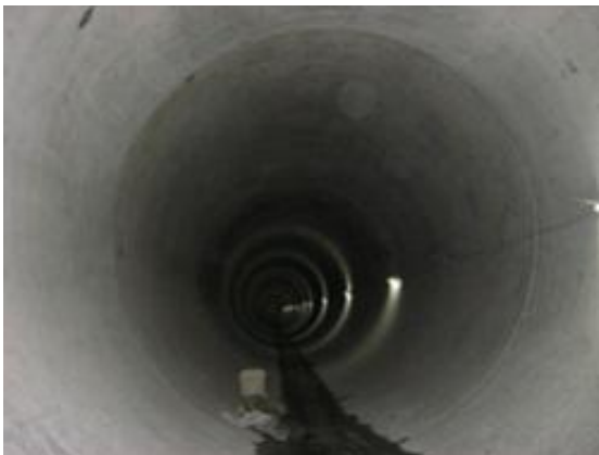
Picture-3 Headrace Tunnel
