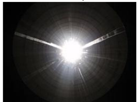
Picture-4 Surge Tank (from the bottom)
