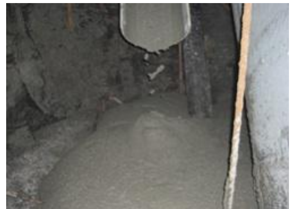
Picture-10 Condition of Concrete at Casting Place
