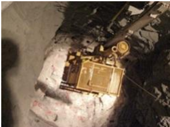
Picture-5 Penstock (Pilot Tunnel)
