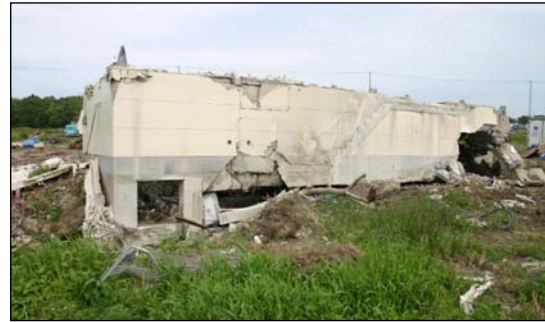
Shichigahama CO building carried away 500 m by the tsunami
