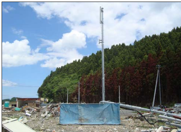
KDDI Cell Site Rebuilt
