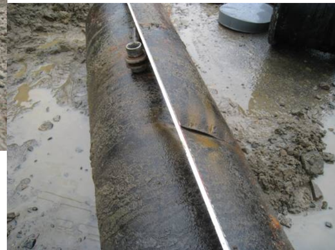
Crack on pipe body
