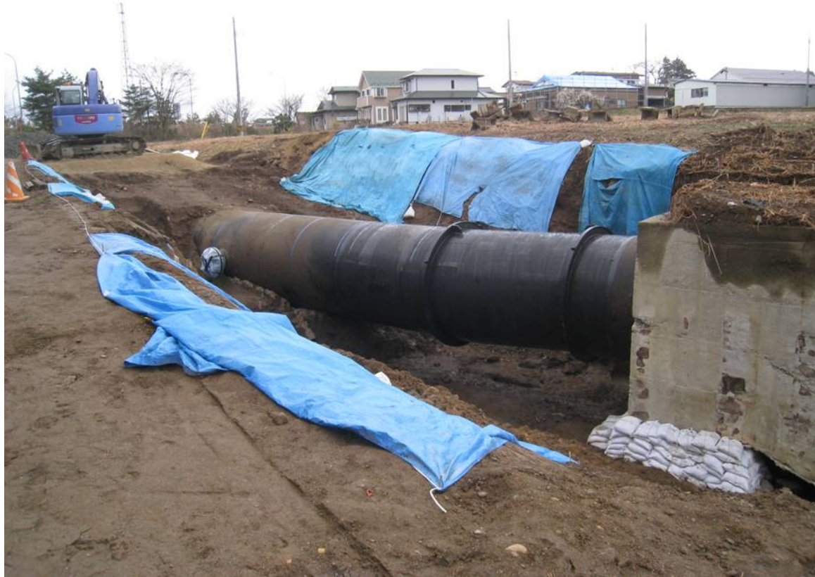
River under-passing transmission pipeline SP \phi 2400
