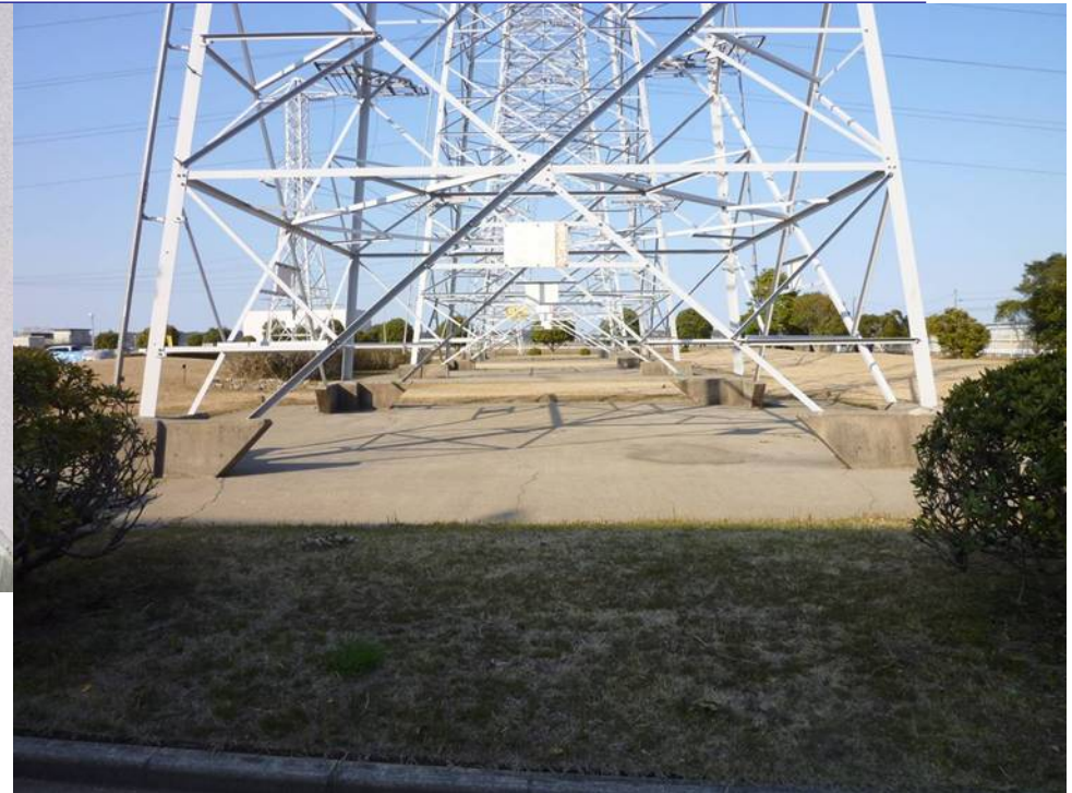
Foundation of Electric power
