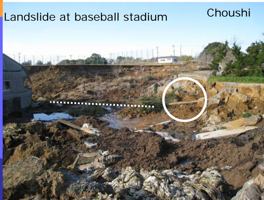
Pipeline damage, DIP \phi 150, due to landslide
