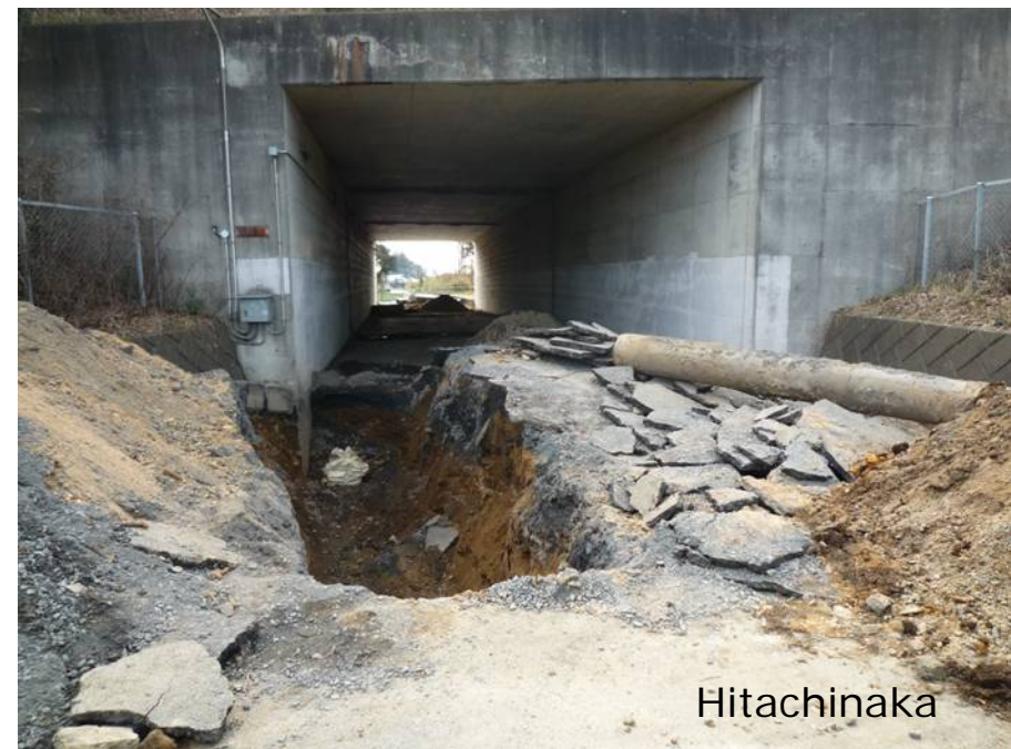
Pipeline damage, DIP(A) \phi 350, due to raised ground surrounding underpass of highway embankment
