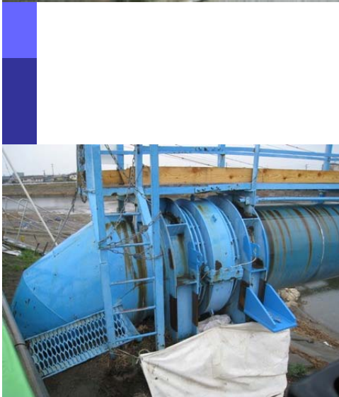
Bearing of water pipe bridge Osaki
