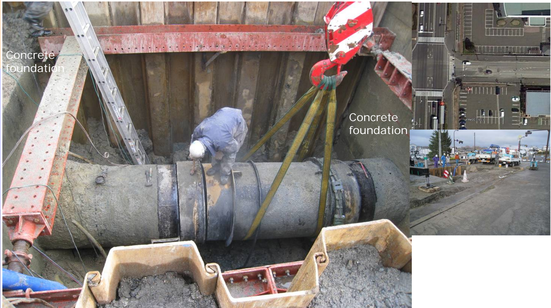
Joint at SP \phi 1200, damaged by April 7, aftershock
