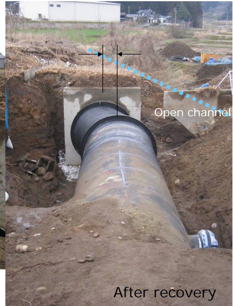
After recovery Lateral sliding 70 cm
