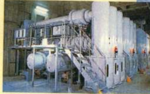
Substation facilities 変電設備
