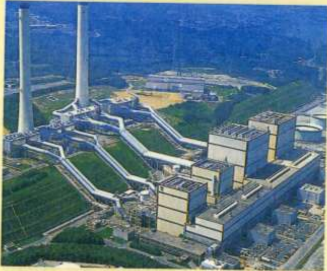
Power plant buildings 発電所建屋
