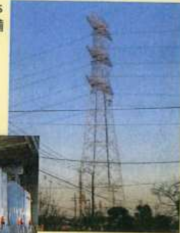
Power transmission facilities 送電設備
