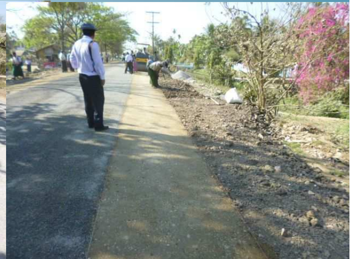
Unloading of materials
