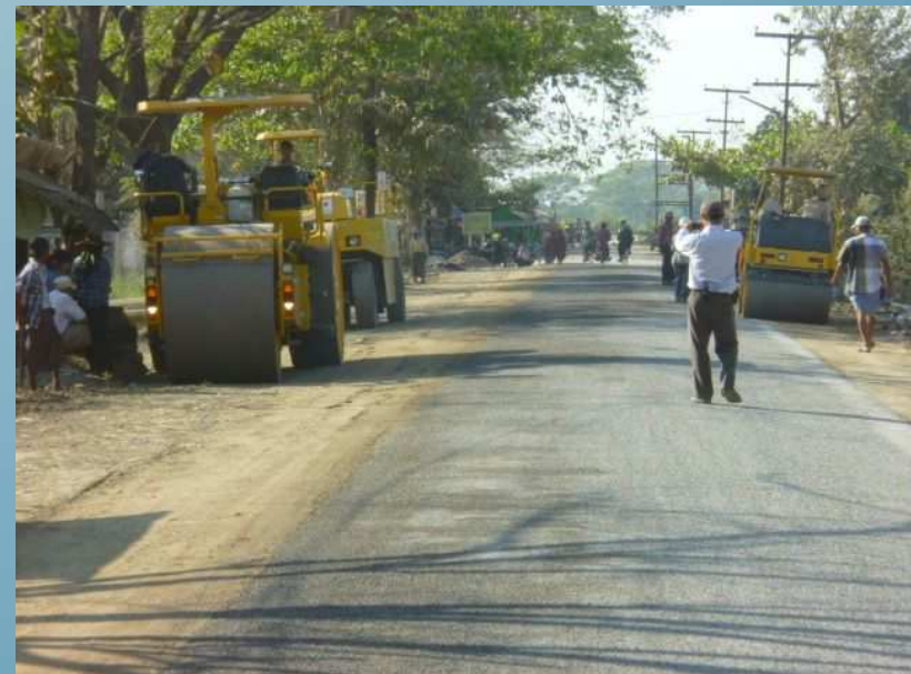
Compaction with a tandem roller
