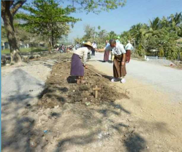
Spreading for shoulders
