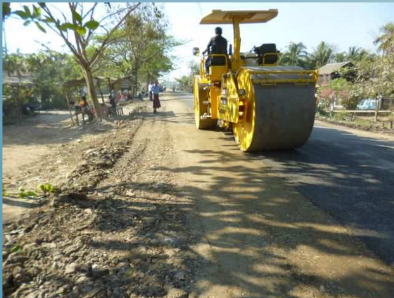
Compaction with a tandem roller
