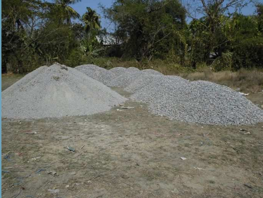
Graded materials for base course
