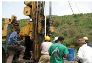
Drilling technology for settlement of a clinometer
