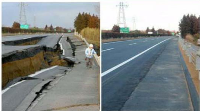
A road in Naka, Ibaraki prefecture, Japan: left, how it was on the day of the earthquake; right, six days later (17 March) after rapid repairs. Photograph: AP
