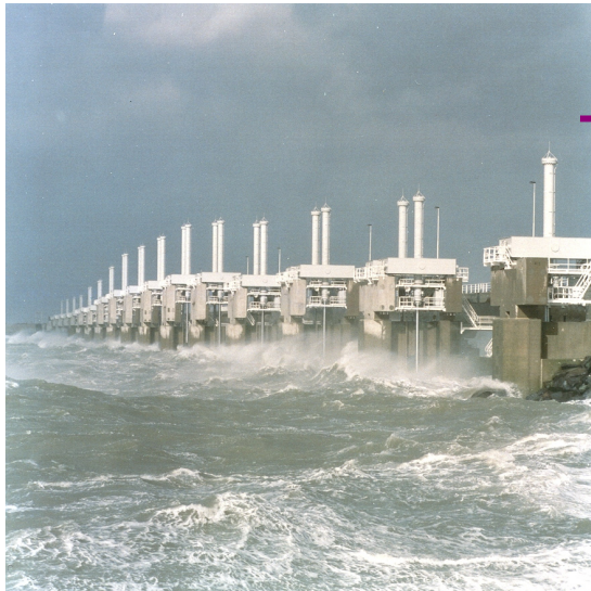
Storm surge barrier in the Eastern Scheldt
