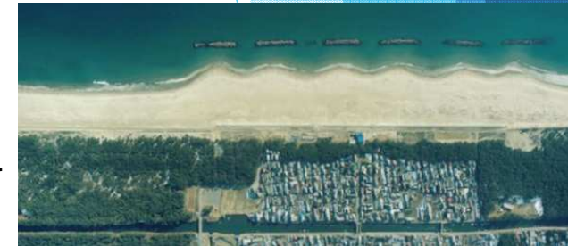
detached breakwater (Arahama Coast, Sendai)
