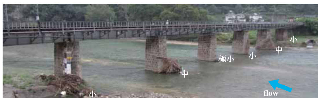
(b) No. 7 (第3三篠川橋梁, 侵食無)
