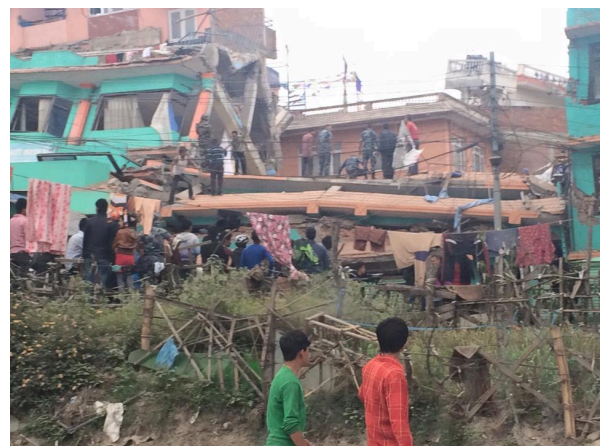
Figure 6 RC framed structure collapse in Kathmandu
