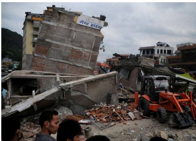
Figure 3 RC framed structure collapsed
