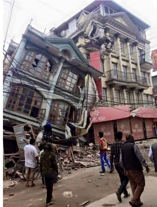
Figure 9 RC framed collapse in Kathmandu
