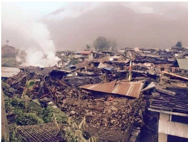
Figure 8 Stone masonry buildings collapsed in Gorkha about 90% collapsed
