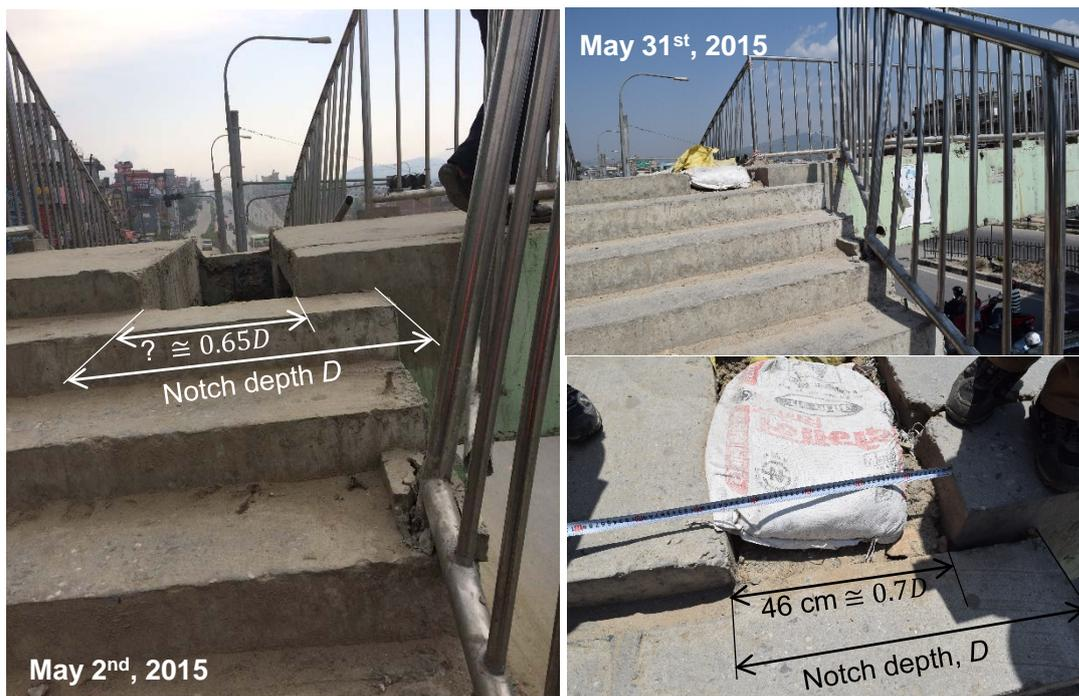
Fig. 11 Joint opened between deck and pier of the pedestrian overpass. Photos left and right by R. Pokhrel on May 2<sup>nd</sup> and 31<sup>st</sup>, 2015, respectively, at N27.674601°, E85.364705°:
