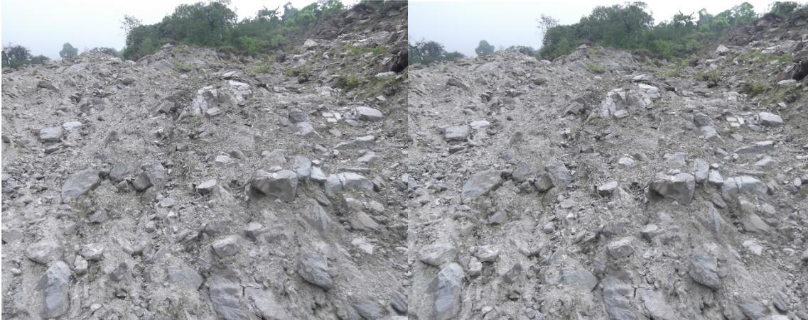
Fig. 8 Sign of dilating debris mass halfway up on a landslide mass, which was cut at this elevation for the temporary road construction at N28.067959°, E85.228808°
