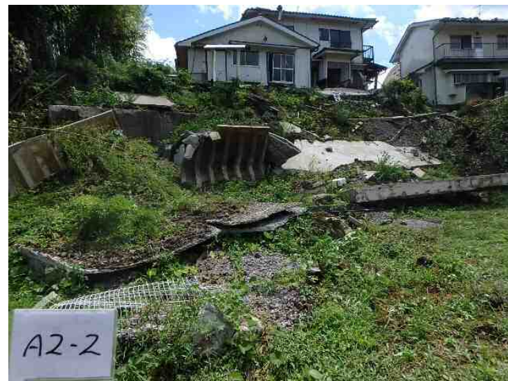
(h) L型擁壁の倒壊 (南阿蘇村)
