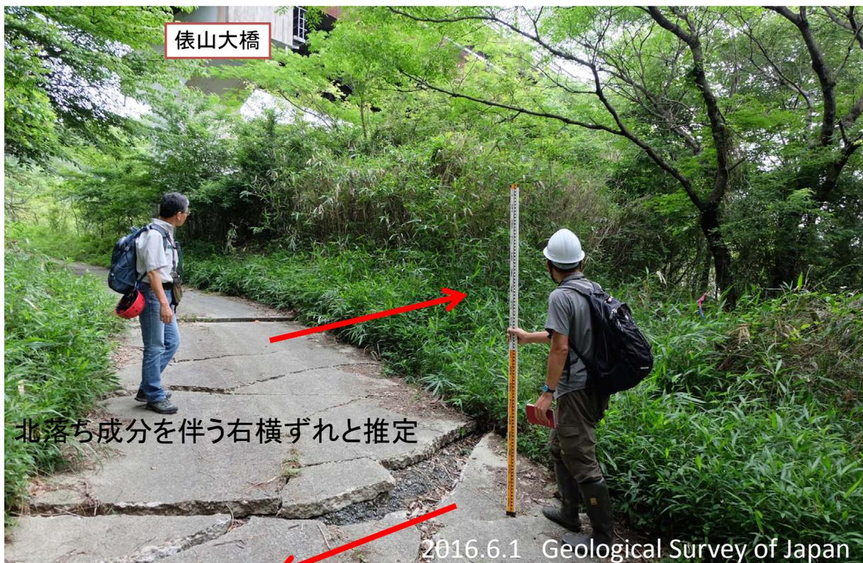
俵山大橋を横切る断層の現地写真(橋上から)
