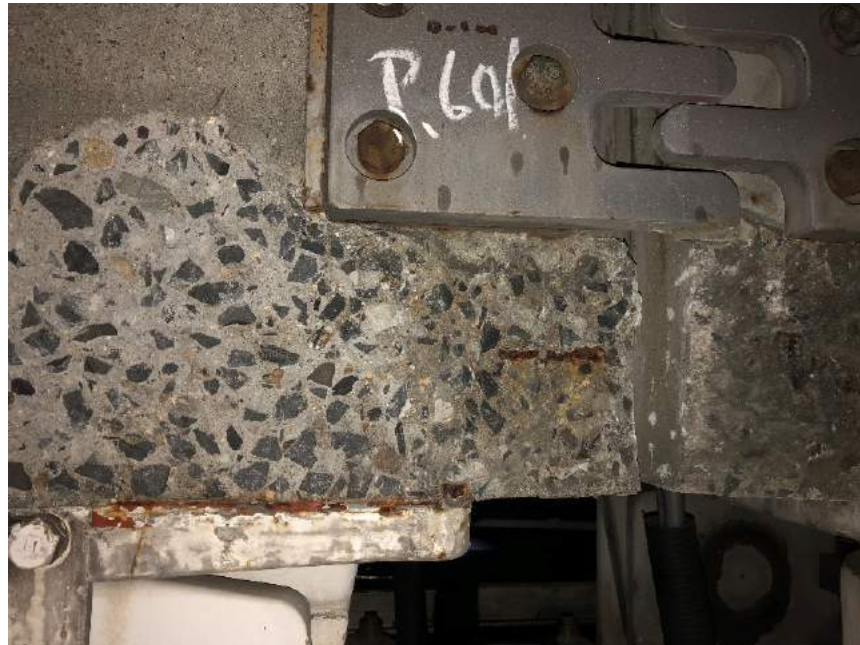
桁側面欠損
