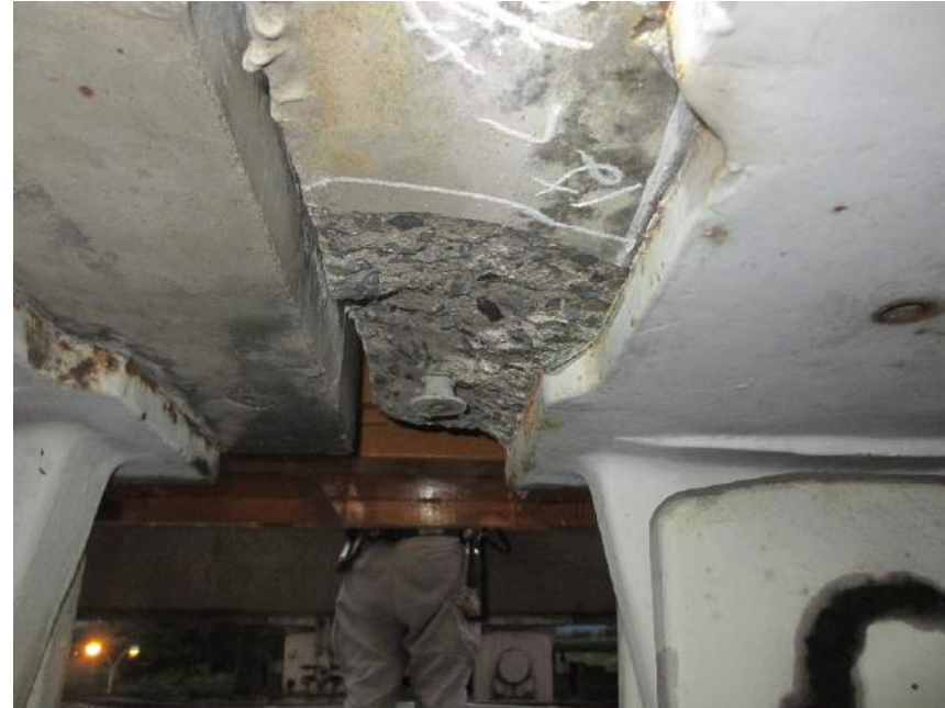
桁下面欠損
