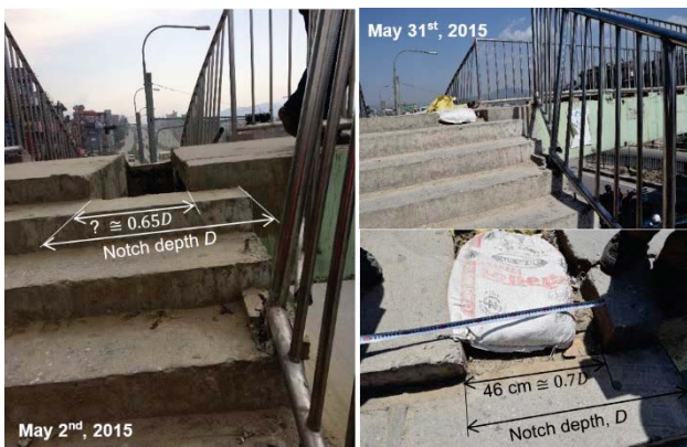
Fig. 11 Joint opened between deck and pier of the pedestrian overpass. Photos left and right by R. Pokhrel on May 2nd and 31st, 2015, respectively, at N27.674601°, E85.364705°: Assuming that the notch depth D of the pier-top landing for the bridge-girder seating is the same for both photos of May 2nd and May 31st, these photos are suggestive that the joint has opened a little wider over a month's period.
