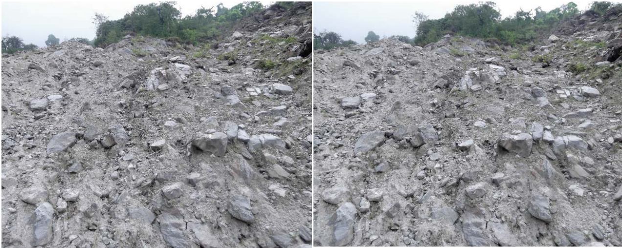
Fig. 7 Sign of dilating debris mass halfway up on a landslide mass, which was cut at this elevation for the temporary road construction at N28.067959°, E85.228808° (Photo by K. Konagai)
