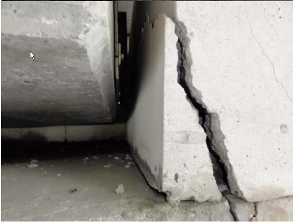
Photo 4 Damage to Suhama Bridge (N34.347940, E134.896113, April 23, 2013)
