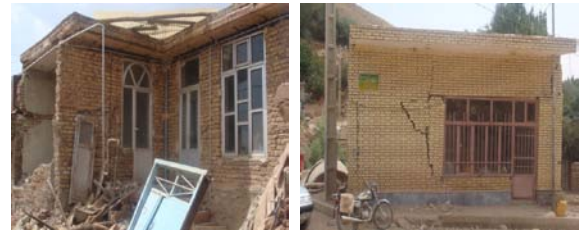
Photo.2 Damage to brick buildings
