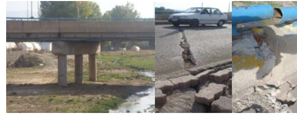
Photo.7 Damage to 6-span composite bridge (No.2)
