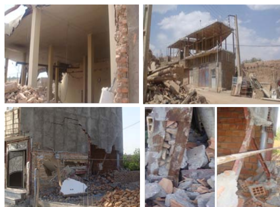
Photo. 5 Damage to steel buildings
