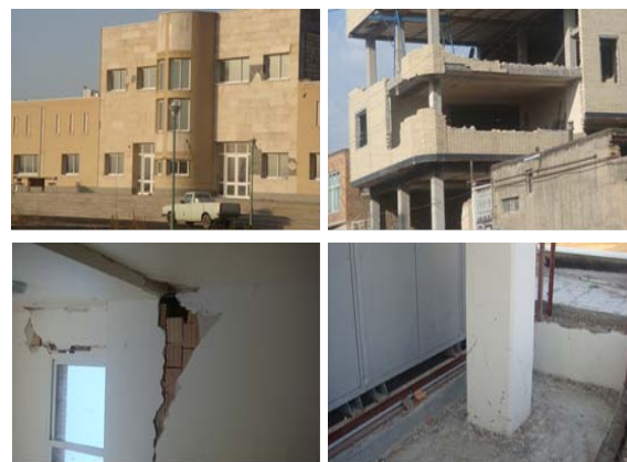
Photo. 4 Damage to reinforced concrete buildings
