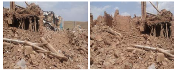
Photo.1 Damage to adobe buildings
