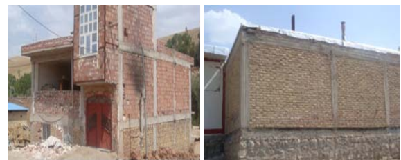
Photo.3 Damage to half reinforced masonry buildings
