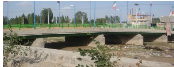
Photo.8 3-span integral composite bridge (No.3)
