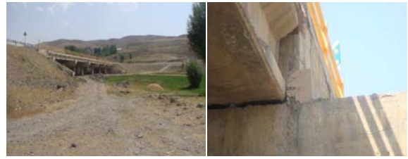
Photo.6 Damage to 5-span concrete bridge (No.1)
