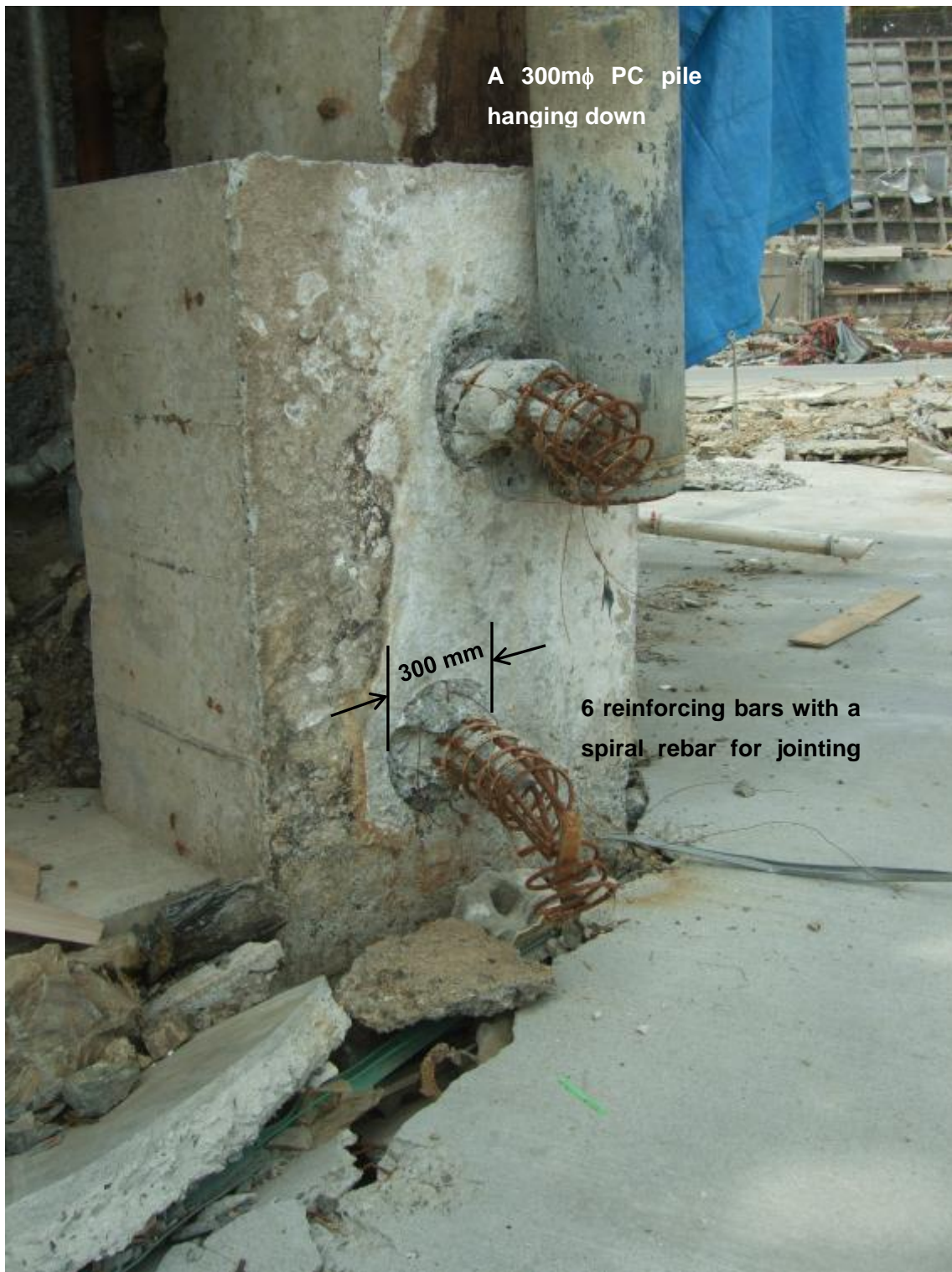
Fig. 6 Detail for jointing pile heads for Building #3: Detail of rebars for jointing a pile head was exposed. There are 6 rebars coiled in a spiral bar for each pile head.
