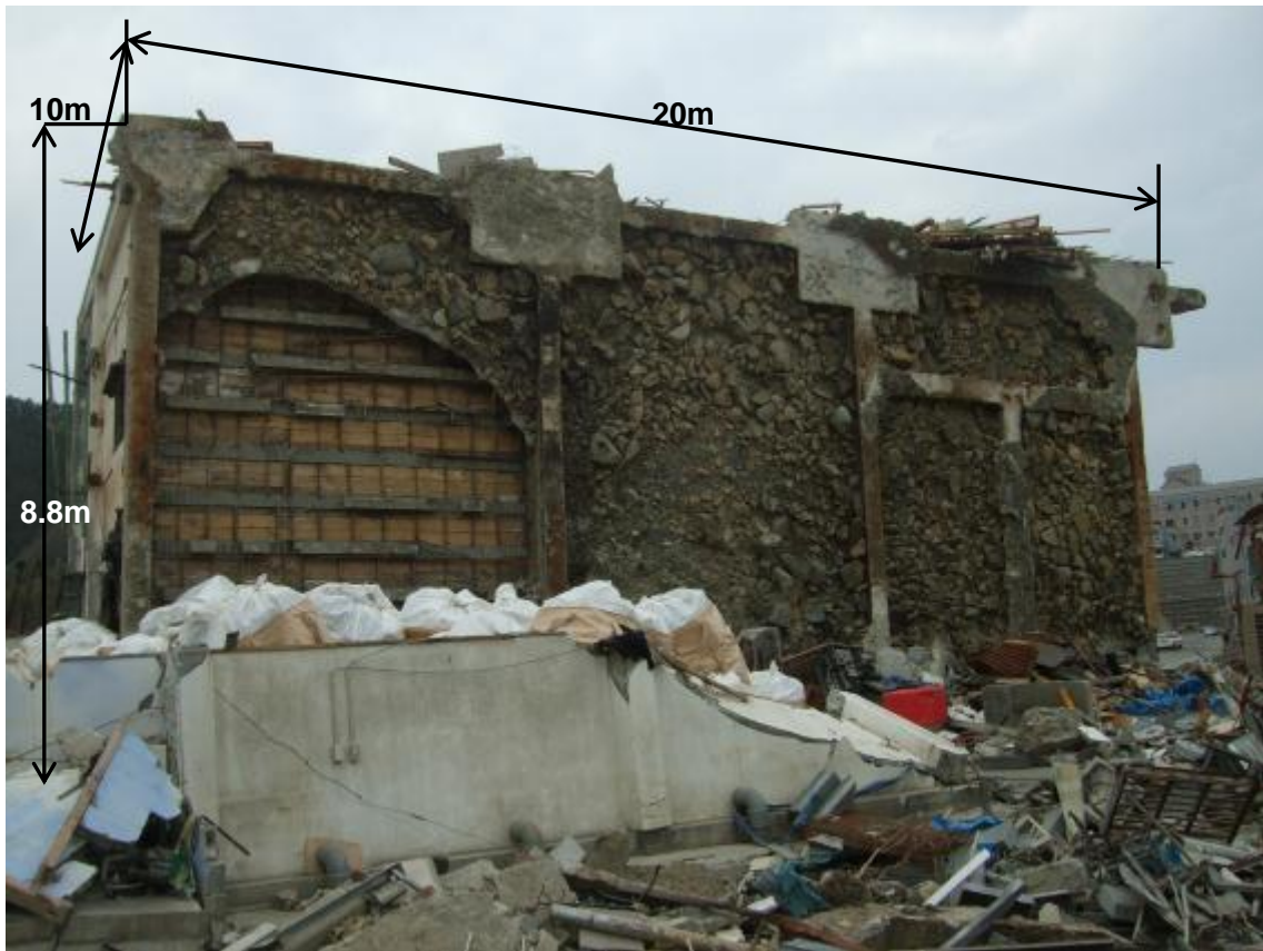
Fig. 7 Building #4: toppled west from its original Location at N38.440608, E141.446511. This was a steel-frame cold storage warehouse for fishes and seafood products. Dim marks of pile head are seen indicating the building was just resting on piles. This warehouse had a small door/window aperture.
