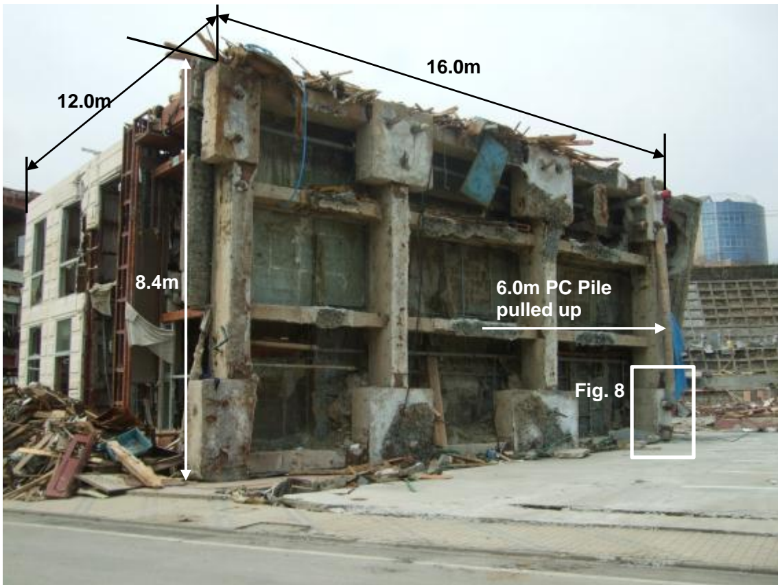
Fig. 5 Building #3 (Original location at Original Location: 38.442657,141.446590), A steel frame 4-story building was toppled and carried sideways over about 20m distance. A PC pile of about 6m long is found hanging down from the upper right corner.
