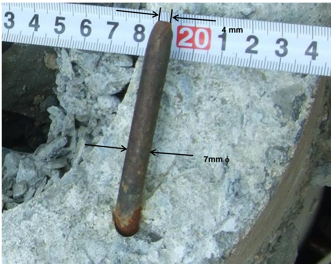
Fig. 4 Fracture surface of PC pile for Building #1: A fracture cross-section of PC (Pretension type centrifugal pre-stressed concrete) pile used for Building #1, 300mm and 120mm in outer and inner diameters respectively, has 7 PC wires exposed with cut ends thinning to about 4mm diameter.
