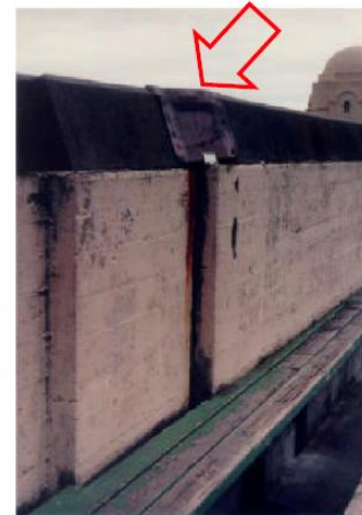
A. Right-lateral displacement of stadium parapet at expansion joint between Sections K-KK (south end of stadium).
