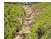
3 Upstream Area with Check Dams
