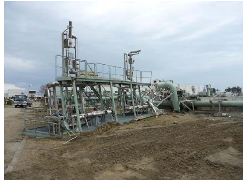
Machinery damaged by tsunami (Tagajoh City)
