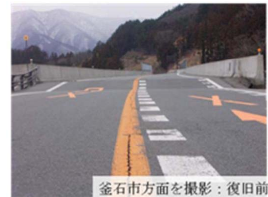
Settlement of approach
