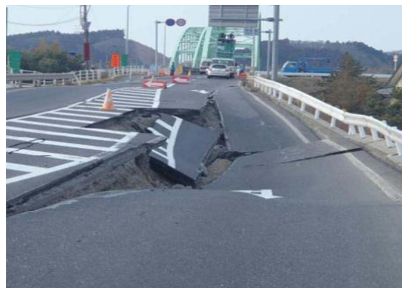
Collapse of embankment
