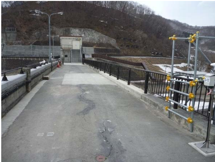
2011 Great East Japan Earthquake
