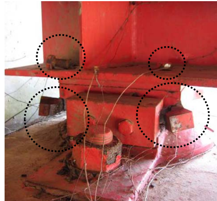
Damage of fixed bearing
