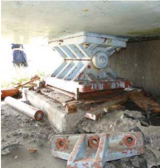
Subsidence of deck end resulting from broken movable bearing
