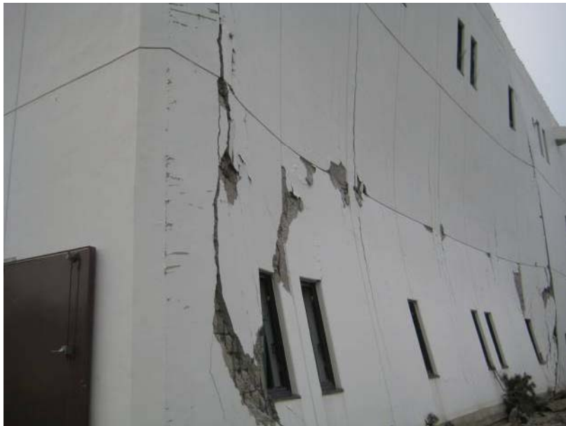
Pumping plant damaged by tsunami (Sendai City)
