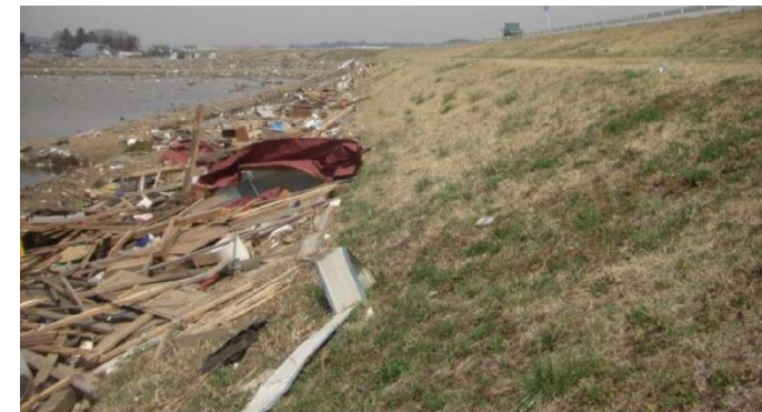
Toe of inner slope
