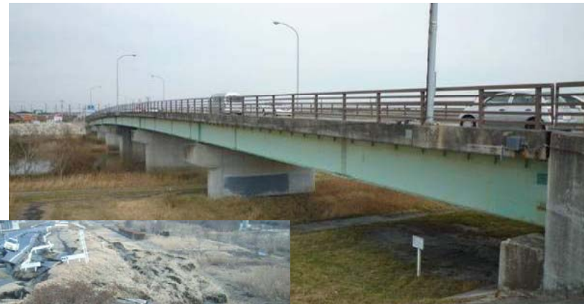
Effects of liquefaction
