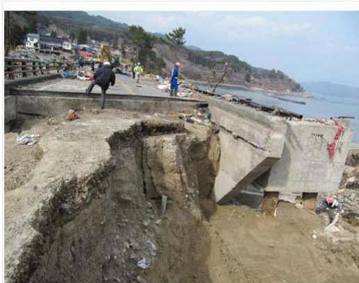
Wash out of embankment
