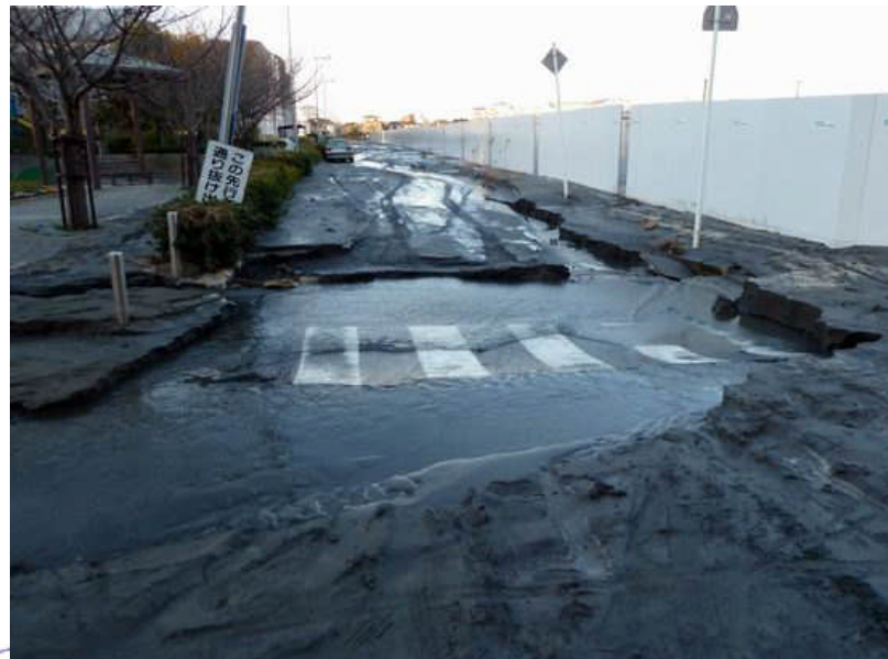
Sand boil and settlement of houses
